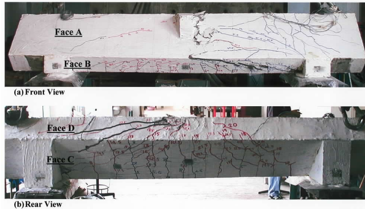
Figure 5. Failure crack pattern of the specimen subjected to bi-axial shear only (Hansapinyo et al. , 2001)
