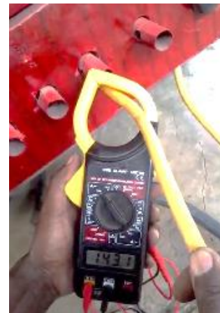
Figure 7. Measurement of the output parameters using a digital clamp multi-meter
