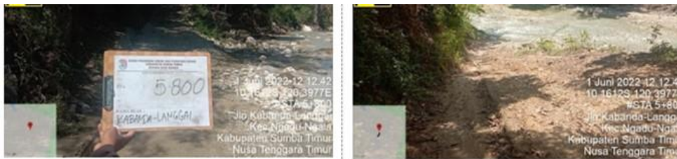
Figure 4. Road link of Kabanda - Langgai STA 5.800, subdistrict of Ngadu Ngala
