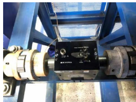
Figure 8. Torque transducer installed in single dynamometer shaft
